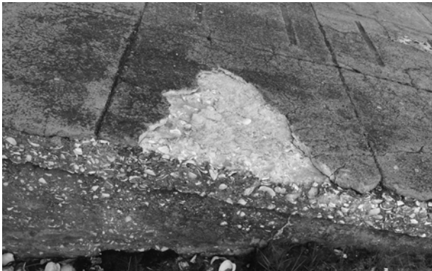
FIGURE 56. View of deterioration on ramp to small boat-room door. (T. Jones, NPS, 2005)
