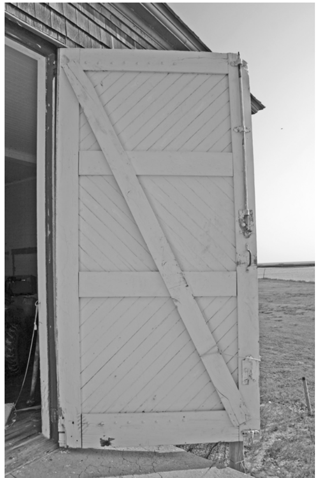
FIGURE 82. View of one leaf of Boat Room door D-3. The diagonal brace is not an historic feature. (T. Jones, NPS, 2005)
