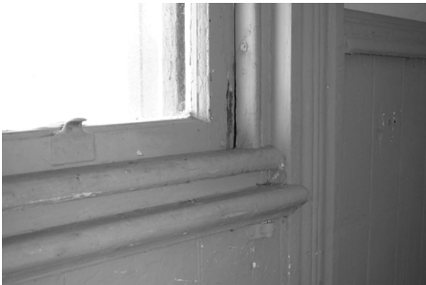
FIGURE 107. View of typical double window stool. (T. Jones, NPS, 2005)
