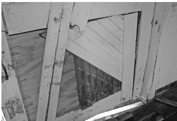
FIGURE 84. View of damage to lower panel of leaf of Boat Room door D-5. (T. Jones, NPS, 2005)
