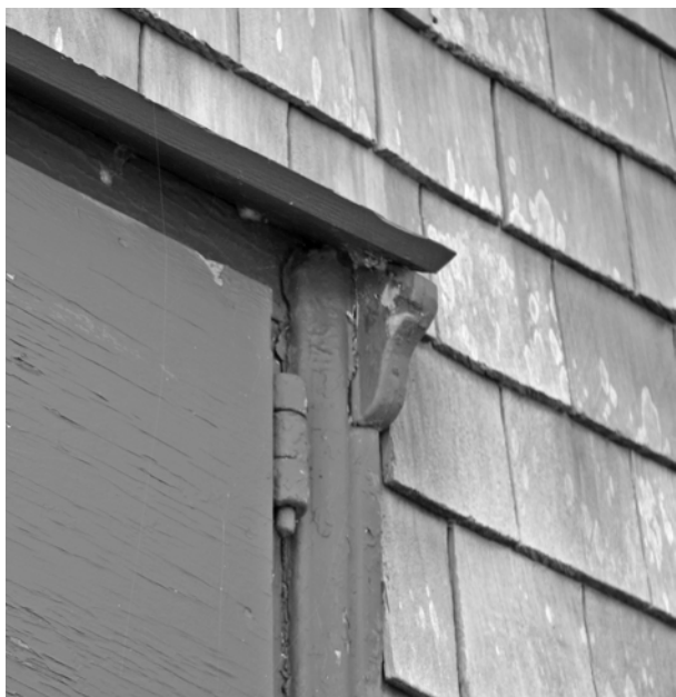
FIGURE 86. View of typical drip cap at Boat Room doors. (T. Jones, NPS, 2005)
