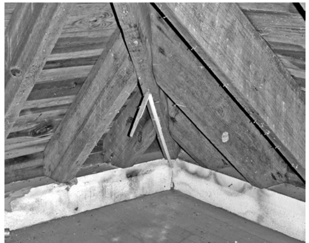
FIGURE 65. View of roof hip and junction of rafters and top plate of second floor walls. (T. Jones, NPS, 2005)
